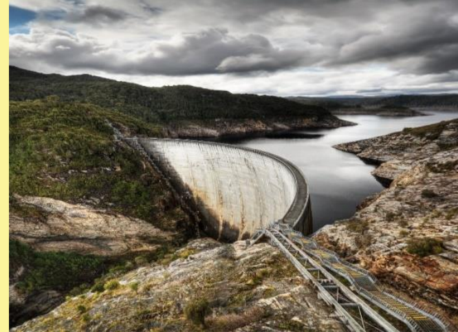
Upstream face of Bhakra Nangal Dam
